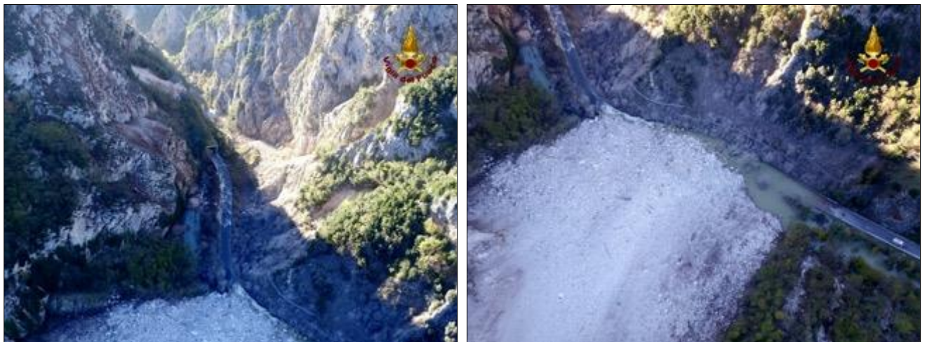
Figure 4.4 The rockfall triggered by the 30 October 2016 earthquake on the sp 209 and Nera river (courtesy of https://www.perugiatoday.it/foto/cronaca/terremoto-norcia-frane-valnerina/aa644aa1.html#&gid=1&pid=1 )
