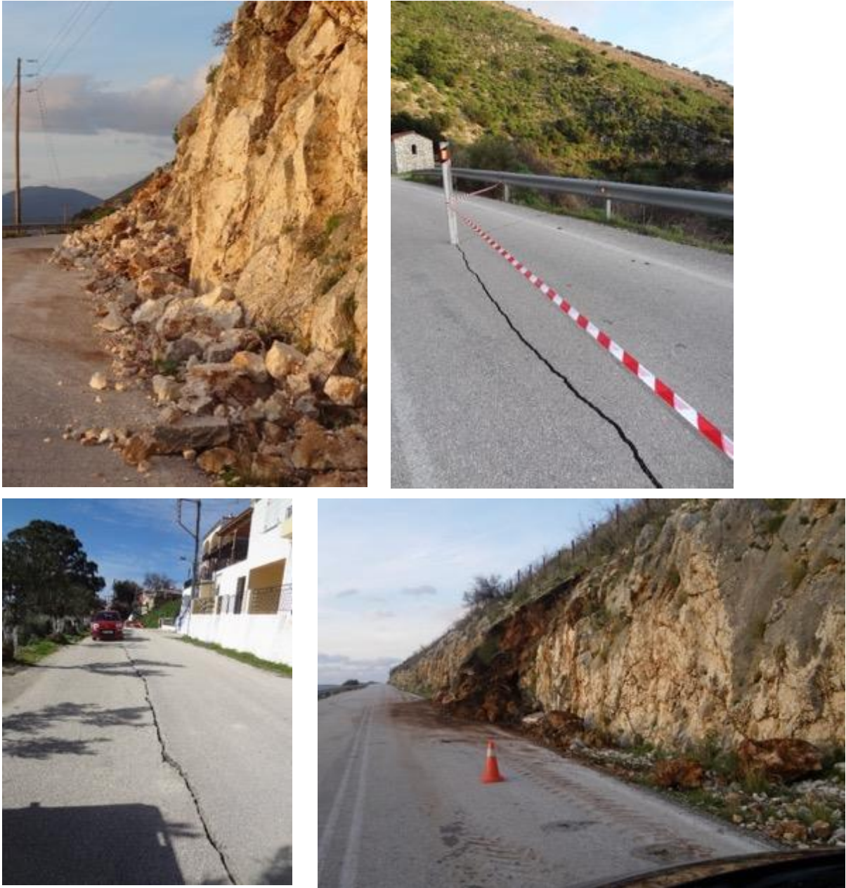
Figure 5.14 Damages recorded along the road network of Ithaca and Kefalonia
