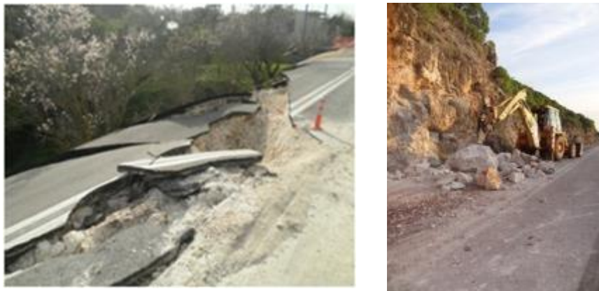
Figure 5.4 Damages on road network (a), landslides and rock falls (b)
