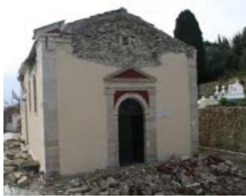
Figure 5.8 Church of St. John in Fafatata, Kefalonia (19th century). Repaired after 1953 earthquake. The outer masonry leaf was severely damaged during the 2014 earthquake. Source: OASP
