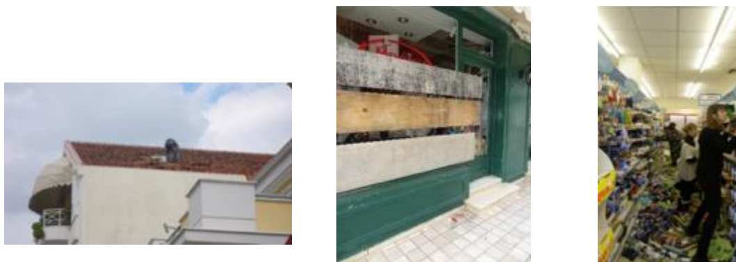
Figure 5.9 Nonstructural Damages (Source: OASP)
