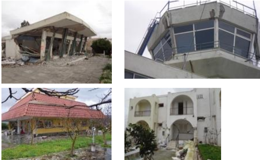
Figure 5.6 Severe damaged structures in Kefalonia
